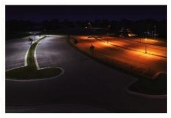
Figure 2. Installation of LED parking for lights (left) compared to HPS lights (right) shows the difference in color appearance and distribution. Photo credit: Beta Lighting.
